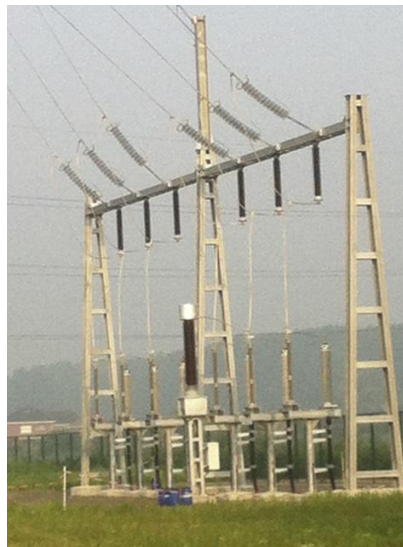
Figure 19. Oil-insulated power voltage transformer application
