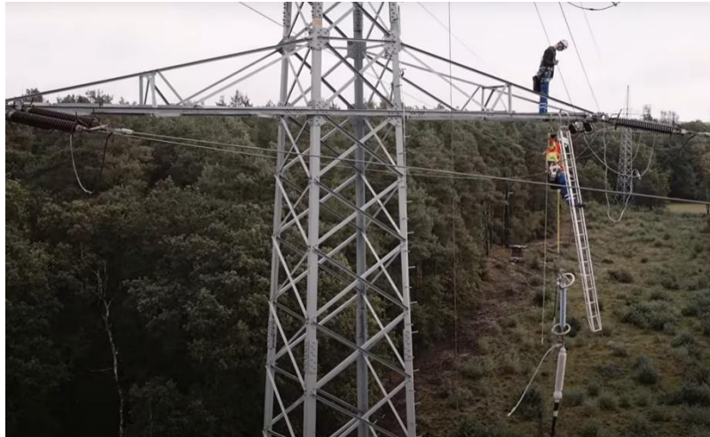
Figure 6. Montage of a temporal cable solution on a 110 kV line [6]
