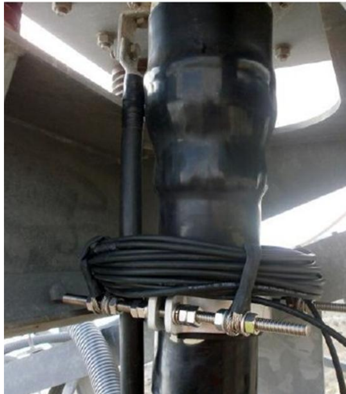
Figure 66. Fibre is wrapped around the cable
