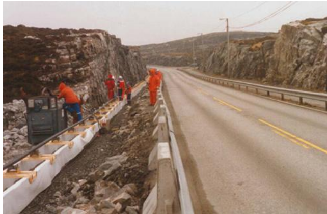
Figure 4. Installation of an existing 300 kV cable
